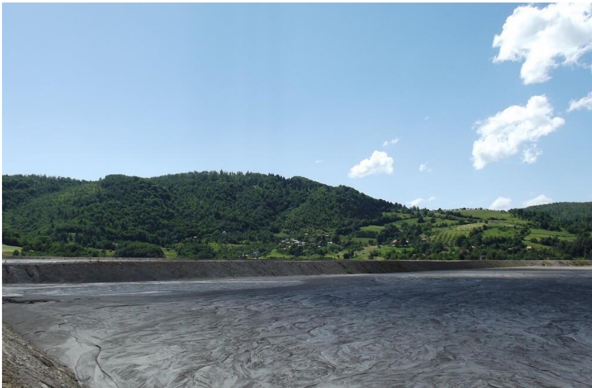
Fig. 1. Zbljevo and Maljevac landfill
