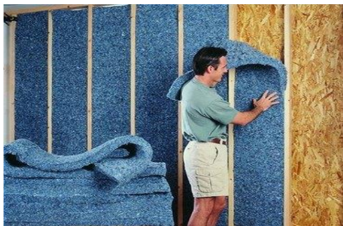
Fig. 3. Recycled blue denim insulation
