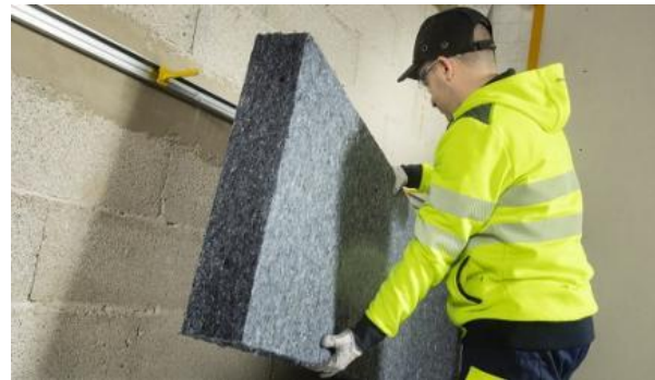
Fig. 2. Recycled textile insulation
