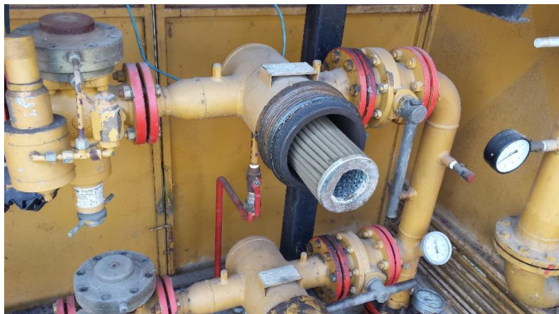
Fig 4. Filter replacement detail
